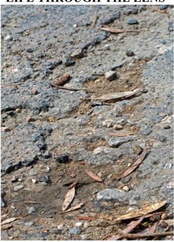
Poor road! There it is! Once shiny and strong! Now cracked; broken with potholes. Wear and tear are taking its toll. Cracks appear allowing water in to undermine the foundation. Weeds take root and cause even more breakdown and damage. Drivers scoff and grumble and declare that this is a useless road. These drivers who once travelled this road now find other roads to use and nobody appears to care. The road is unable to fix itself and continues to crumble.
